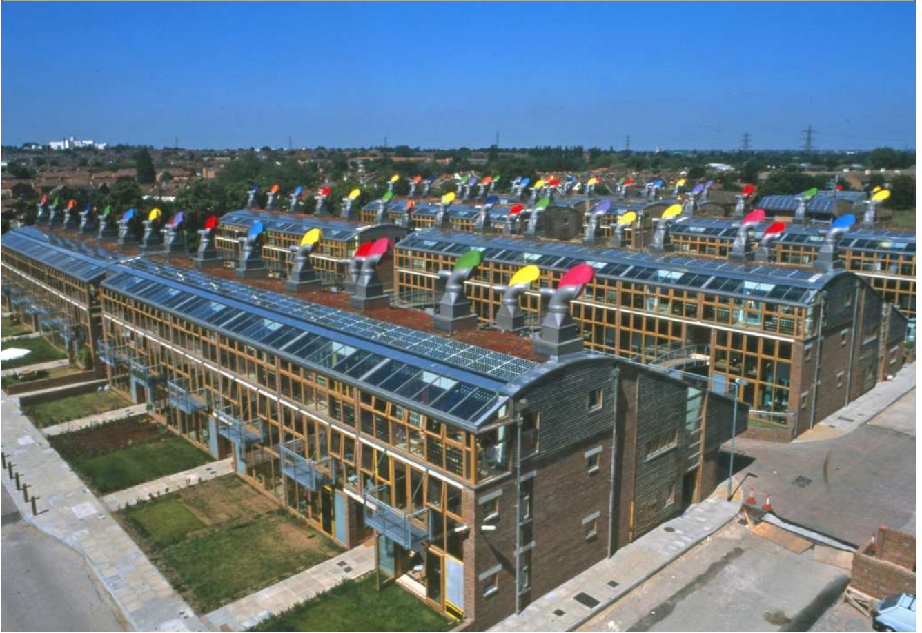
Figure 14: BedZED community development (courtesy of Wikimedia commons) © Arup
