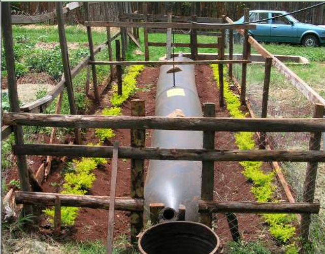
Figure 60: Biogas Generator by Pioneer. Source: © SuSanA Secretariat
