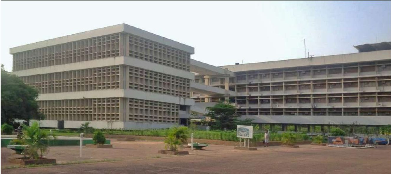
Figure 33: Bioclimatic strategies in typical urban buildings: Shading and natural ventilation.
