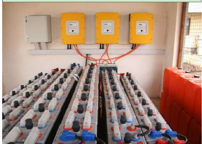
Figure 53: Flooded deep discharge lead-acid battery bank feeding three SMA Sunny Island inverter/chargers. Image Source: © DreamPower Solar.
